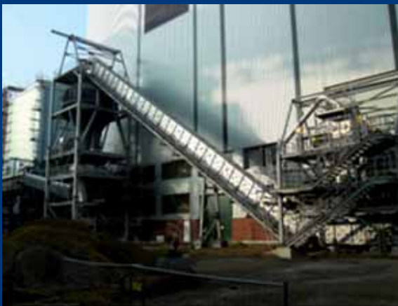
Dry bottom ash handling system at Walsum #10 (Photos: HPE)
