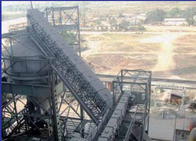
ECO ash conveyor, postcooler and silo in Durgapur Unit #7.
